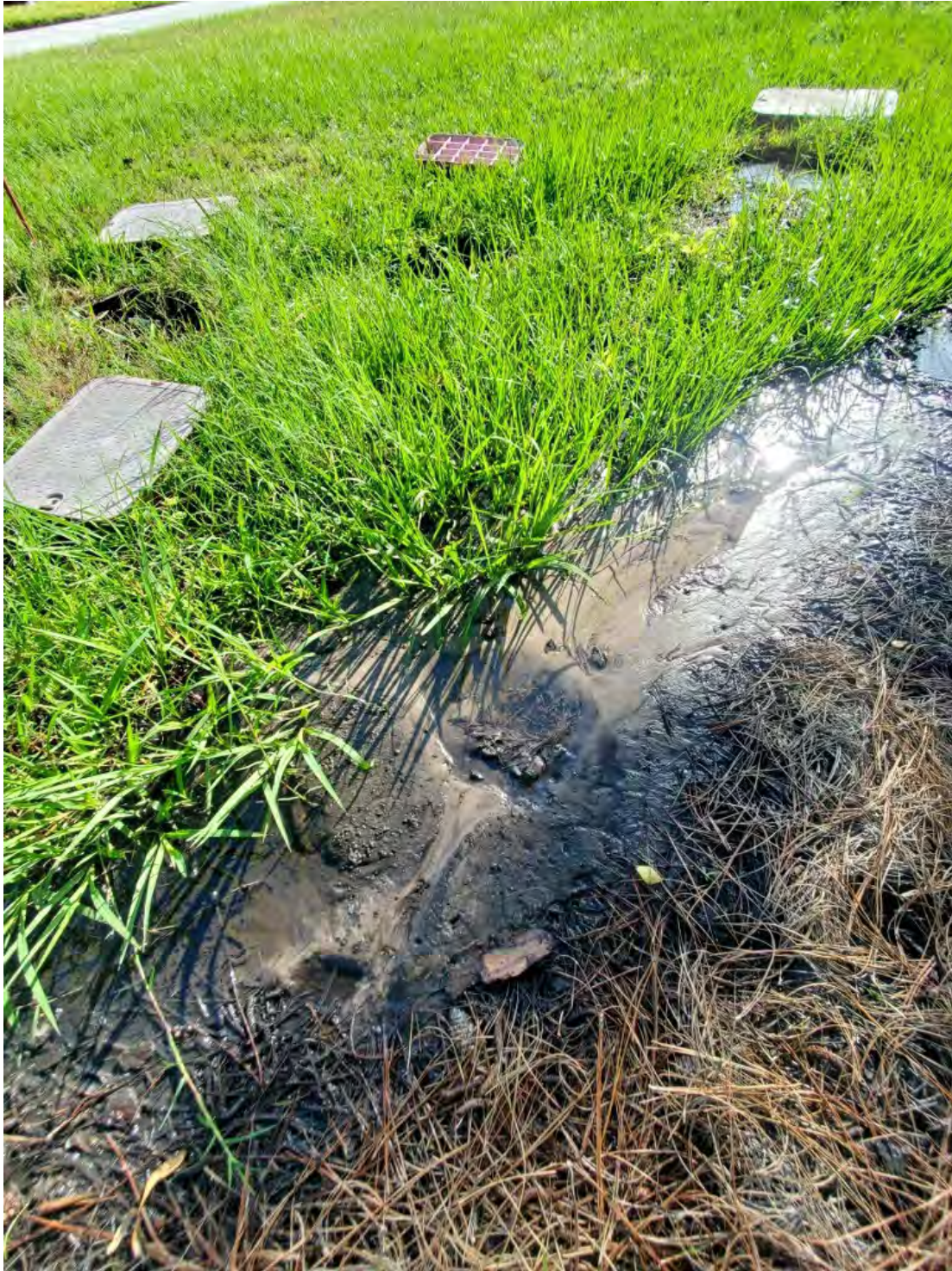
Mainline leak in SW corner of round-about at Connerton Blvd and Bluemist.
